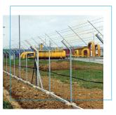
Senstar also offers a taut wire perimeter intrusion detection system. It has no environmental limitations with a very high Probability of detection (Pd) and a virtual absence of false and nuisance alarms. It can be installed on either an existing carrying fence or on a fence specifically designed as a barrier.
