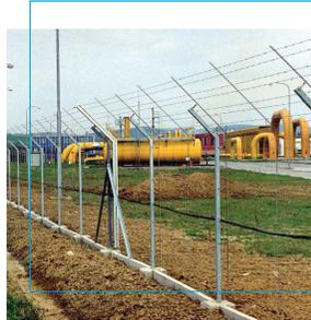
Senstar also offers a taut wire perimeter intrusion detection system. It has no environmental limitations with a very high Probability of detection (Pd) and a virtual absence of false and nuisance alarms. It can be installed on either an existing carrying fence or on a fence specifically designed as a barrier.
